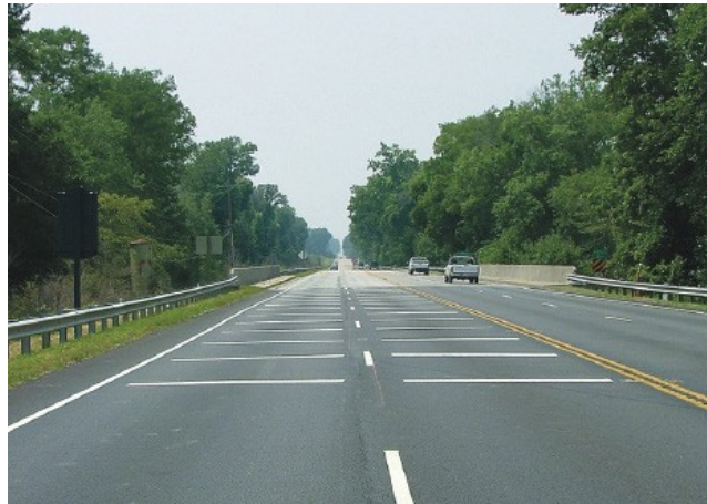
Example of full-lane transverse bars
