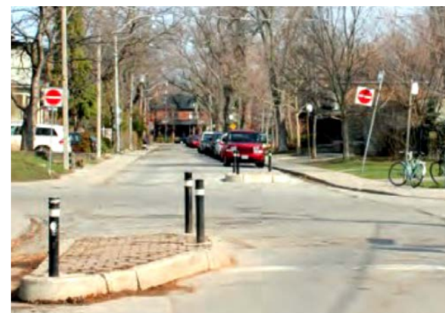
Example of a directional closure sign
