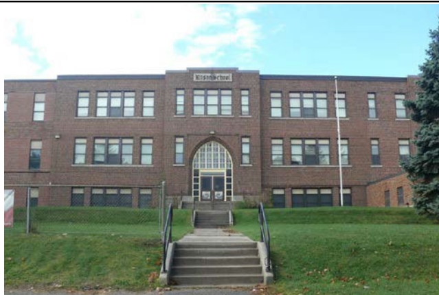
Main Façade (East) – September 2012
